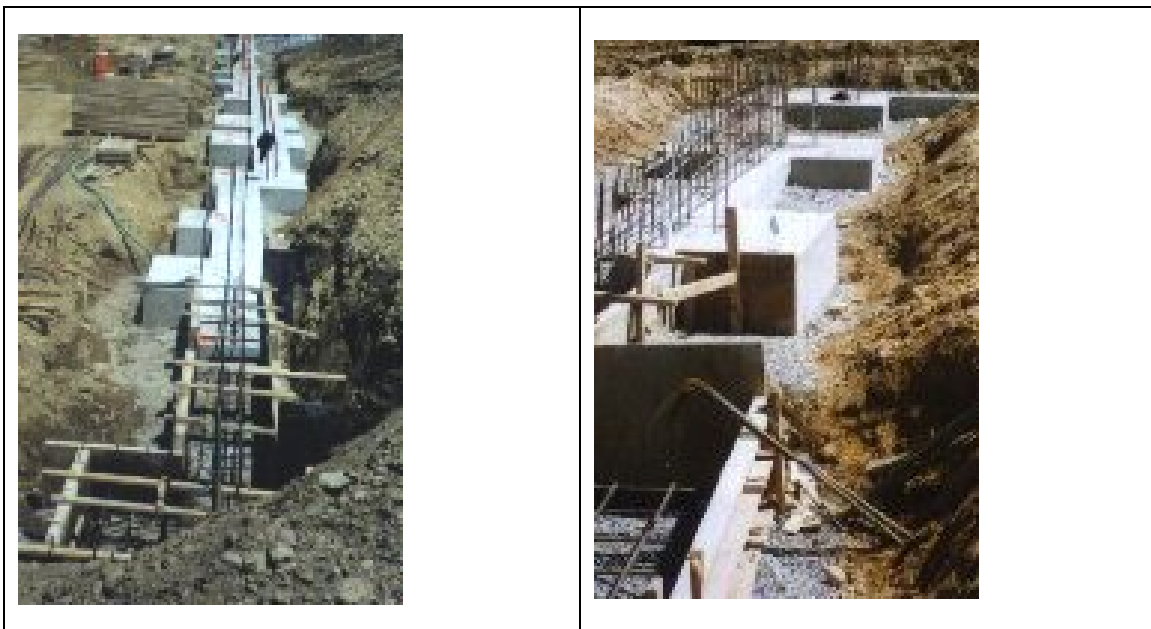
Photograph 4.1 – Shallow Spread Footings
