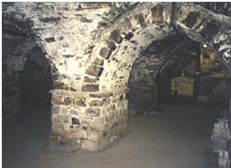
Photograph 1.1 - Foundations for a Medieval Era Cathedral
